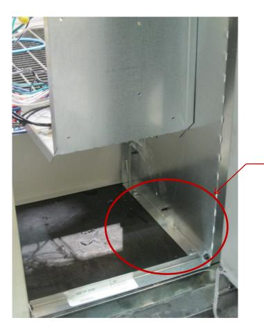
Mounting locations at base of unit (interior view of unit)
