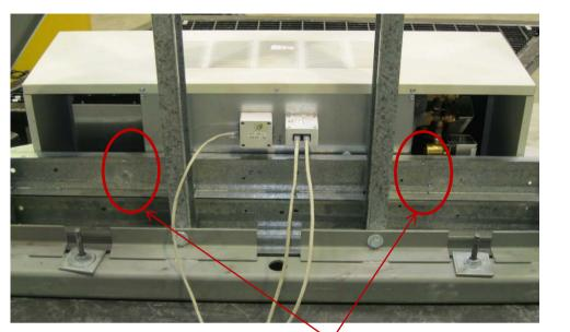
Mounting locations at back of unit (rear view of unit)
